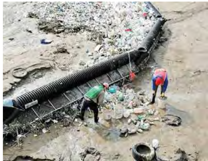
WILD COAST installed a “trash boom” along the Tijuana River to capture and recycle plastic waste. Photo courtesy of WILD COAST.
